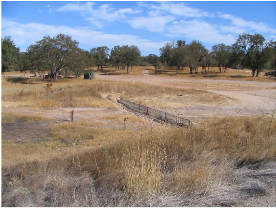
Fish Screen Installation
